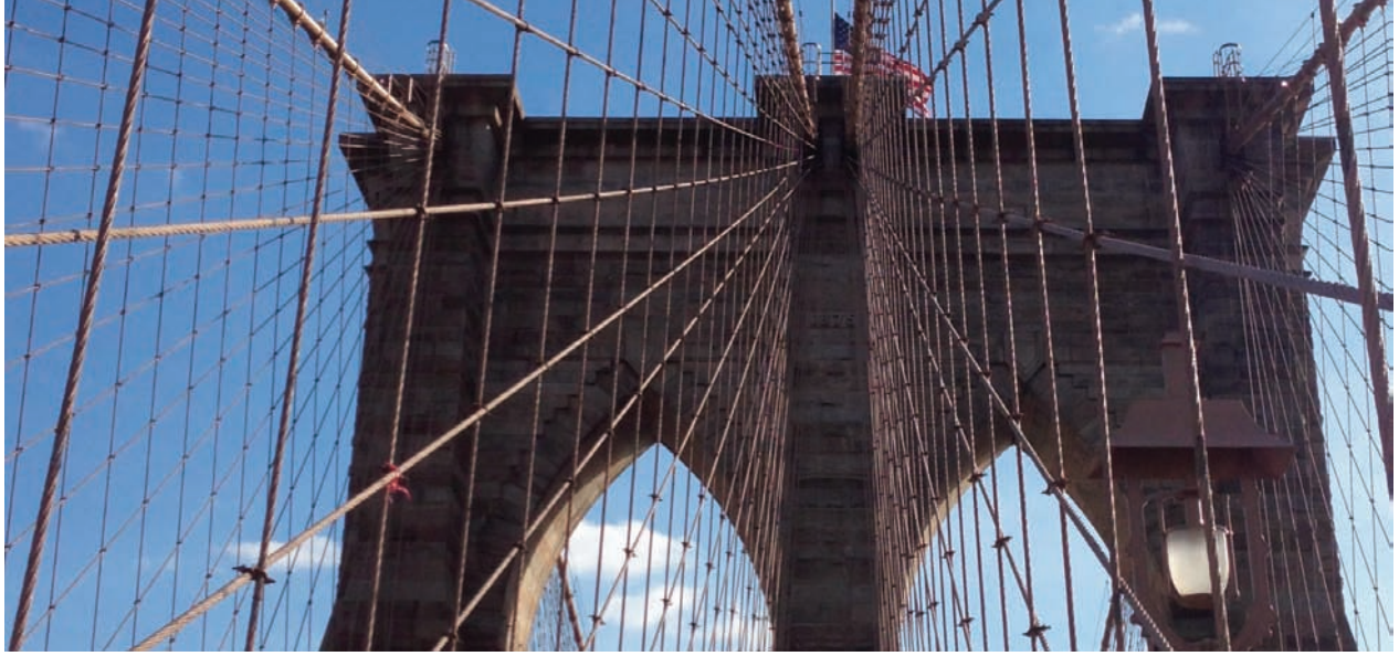
Detail of Brooklyn Bridge. Photo by Randall Stephens.
